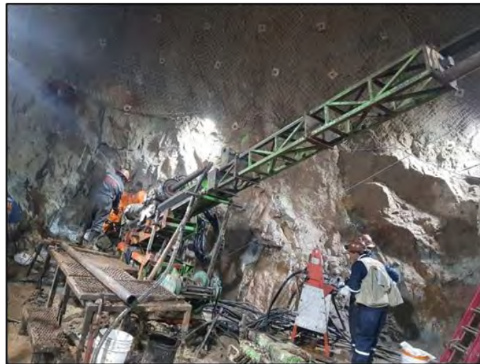
Figure 10.6 Drill Bay at Huayra Kasa Adit
